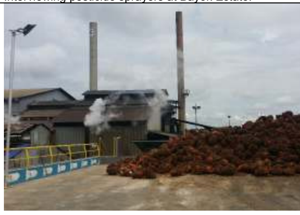
FFB loading ramp at Pamol Sabah POM.
